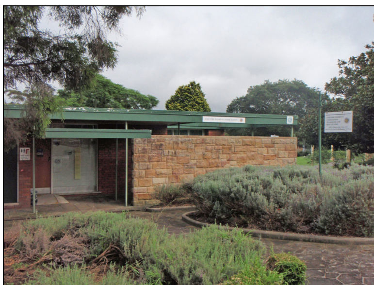
Figure 8: Front elevation of Women's Rest Centre showing sandstone wall to be carefully dismantled and relocated as indicated in the picture above.
